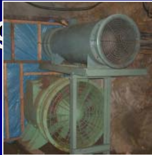
Large fans mounted on the top of shaft to generate and control the updraft velocity
